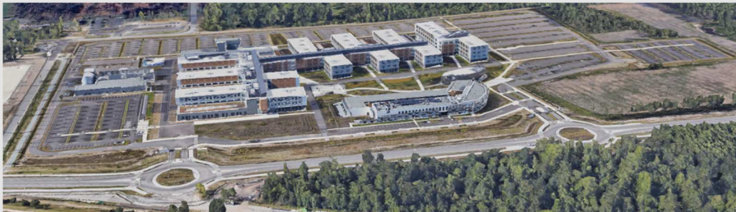
Campus industriel Thales Mérignac (33)
